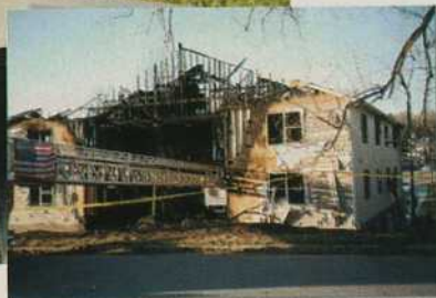
Sarah had to jump to safety from her third-floor apartment. Below, the burned building.
